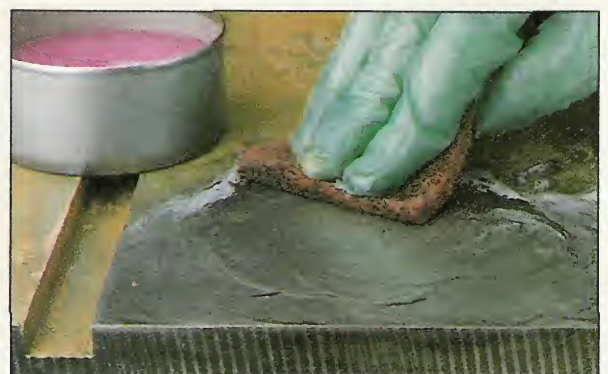
B. Rub in Chemical with Stripping Pad. A combination of a chemical dissolver like Naval Jelly and a furniture stripping pad removes the rest of the rust.
