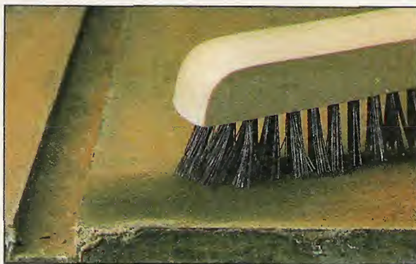
A. Remove Loose Rust. To get a better look at the condition of the top, a wire brush is used to remove most of the dirt and loose rust.
