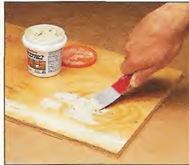
Step 1. First, sand the surface and then fill any cracks and voids. After the filler dries, sand again.
