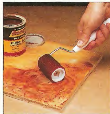
Step 1. After the sanding sealer is completely dry, roll out one or two coats of contact cement.
