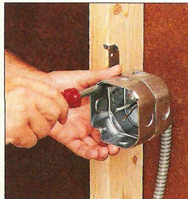
▲ Box Extension. An easier way to extend electrical boxes is with extensions. They're available at most home centers.
