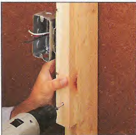
Step 1. Before you begin work on the ceiling or walls, you'll need to extend all of your electrical boxes.
