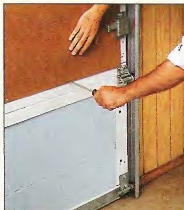
▲ Overhead Doors. You can increase the STC of a garage door by filling the panels with insulation and covering it with Masonite.
