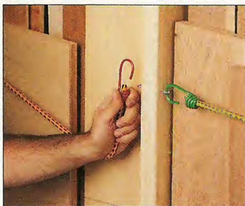
▲ To hold "shorts" in place, I installed screw eyes in the uprights and ran stretch cords across the storage compartments.
