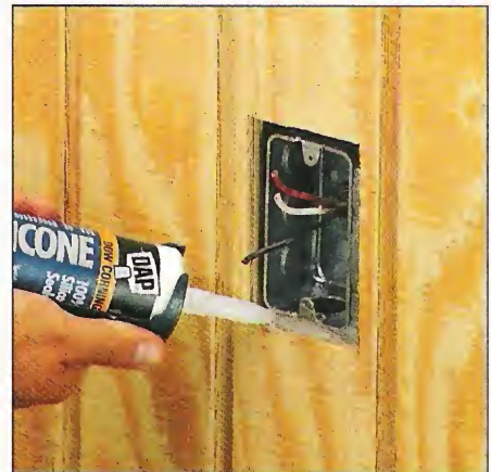
Step 6. To seal noise in, and still allow the walls to flex, fill in any gaps with a high-quality silicone caulk.
