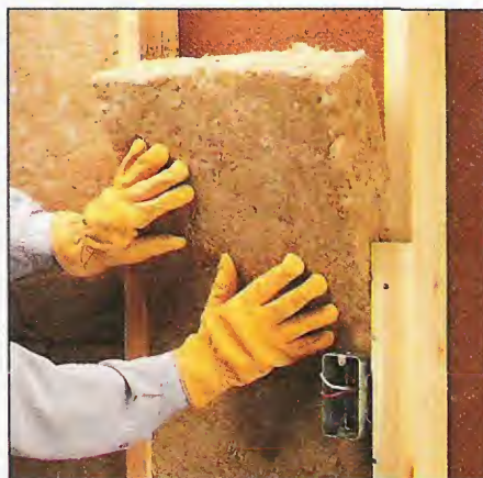
Step 2. A quick and inexpensive way to increase the STC of a wall is to tuck a sound blanket between the studs.
