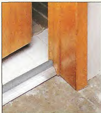
▲ Entry Doors. To help sound-proof a door, install a threshold (or door sweep) and apply weather stripping to the edges.
