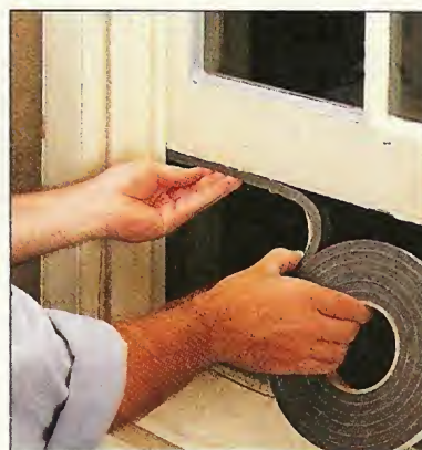
▲ Seal Windows. To reduce the amount of noise passing through a window, install weather stripping around the edges of the window.
