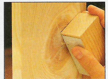
filling all the holes and gaps, allow it to dry overnight before sanding and finishing.
