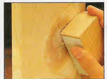
filling all the holes and gaps, allow it to dry overnight before sanding and finishing.
