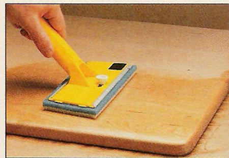
C. Pad. For large surfaces, a paint pad works best. It loads well and lets you apply the finish quickly and evenly.
