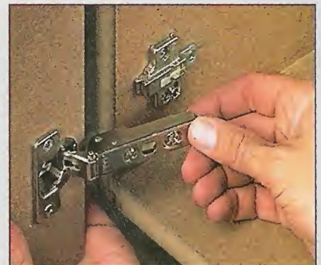
Step 3. To hang a door, just snap the hinge clip on the mounting plate, then adjust the hinges to position the door.
