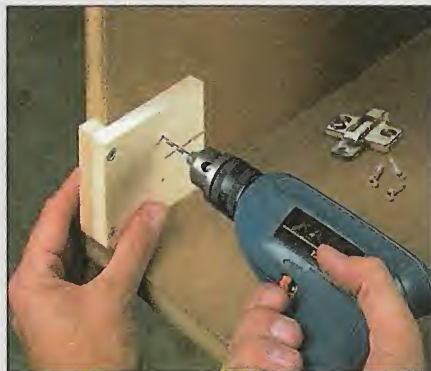
Step 2. Next, drill pilot holes in the side of the cabinet for the mounting plate screws, refer to template above.
