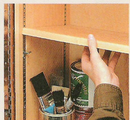
C. Adjustable Shelving. Metal shelf standards allow you to adjust the shelving for your storage needs.
