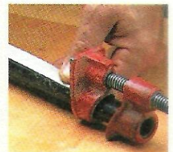
Applying a strip of masking tape to the pipe prevents the iron from reacting with the water in the glue and staining the wood.
