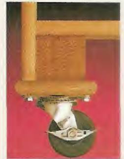
A thick corner block directs the weight of the cabinet and tools onto the casters.
