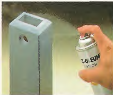
Step 4. Finally, spraying on an acrylic clear coat helps to protect the painted finish.
