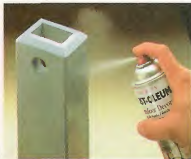
Step 3. To ensure uniform coverage, use a sweeping motion as you spray on the color coat.
