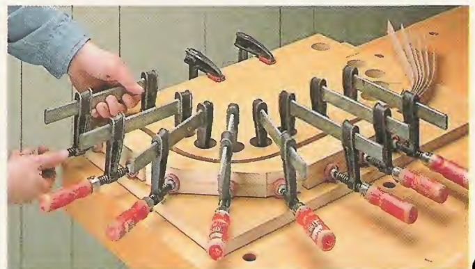
4 After removing the clamp at the end of the form, you can add the last pressure block on the first side. Finally, repeat the process for the other side of the form.
