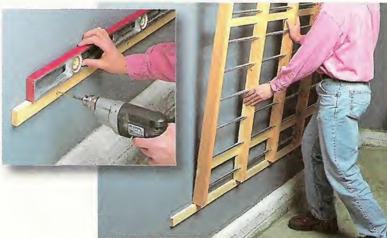
1 A long strip of wood that's temporarily screwed to the wall provides a convenient support as you raise the grid. Just be sure it's level, see inset.
