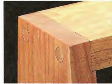
▲ Two Versions. You can use hand-cut dovetail joints (see photo at left) or rabbets, woodscrews, and plugs (right) to hold the rack together. Either way, it creates a strong, mechanical joint.
