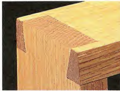
▲ Two Versions. You can use hand-cut dovetail joints (see photo at left) or rabbets, woodscrews, and plugs (right) to hold the rack together. Either way, it creates a strong, mechanical joint.
