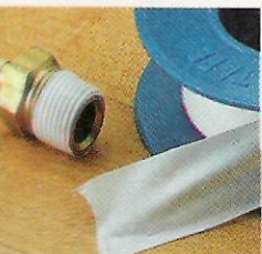
▲ To produce an air-tight seal, wrap the threads of the brass fitting with Teflon tape before screwing it in place.
