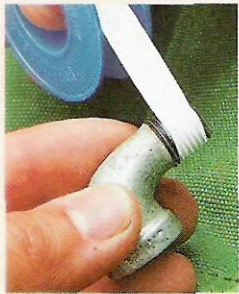
▲ To produce an airtight seal, wrap the threads of the pipe fittings with Teflon tape.
