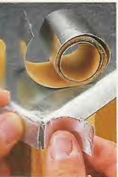
A quick way to cover the sharp edge at each corner of the cover is to stick on a small strip of aluminum tape.
