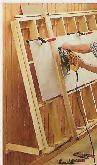
C. Partial Sheets. A row of support blocks holds partial sheets at a convenient height.
