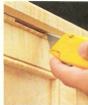
▲ To lay out the location of the hinge on the lid, simply score a line using the mortise in the chest as a guide.
