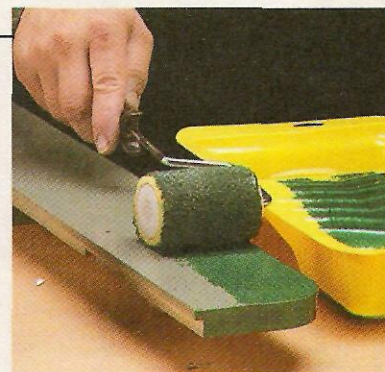
Step 2. After covering the edges, roll the paint on the faces, making sure to lay down a good, “wet” coat.
