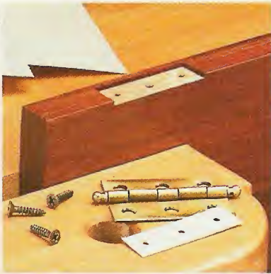
▲ To shim deep hinge mortises, Bob Britzke of Eureka Springs, AR uses 1/64" model airplane plywood, available at hobby stores.
