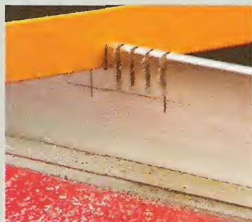
▲ Cut. To create the notches for the T-track, start by cutting a row of kerfs with a hack saw.
