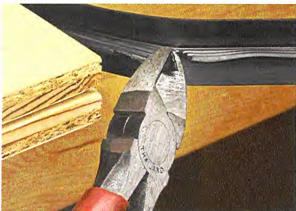
▲ Notch It. Fitting the molding around a 90° corner requires a notch. I used flush-cutting pliers to cut a small V-shaped piece from the barbed section.
