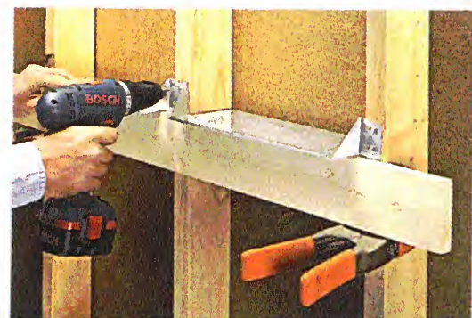
▲ Aligning Multiple Shelves. Clamp and level a straight 1x4 across several studs to quickly install a line of these shelves.
