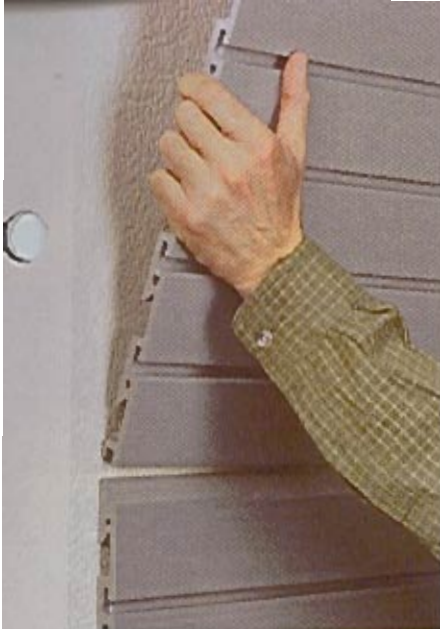
▲ Interlocking Panels. The interlocking feature makes installing multiple panels easier.
