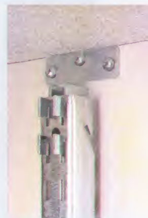
▲ T-Bracket. The T-bracket screws securely into a stud or along the top plate of your wall.
