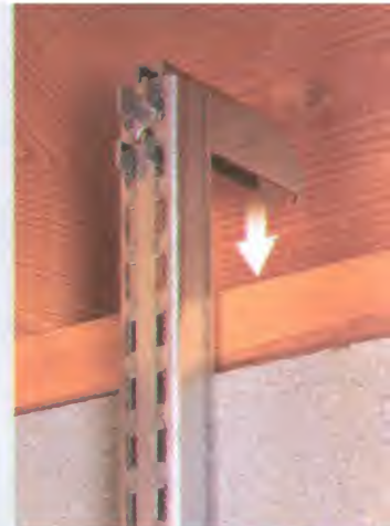
▲ Hook. If your ceiling is unfinished, you can hang the uprights from the top plate using the hooks.
