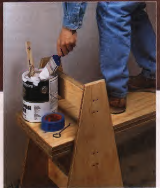
► Mini-Scaffold. By placing the plank on one of the lower stretchers of the sawhorses, you can use it as a platform when you need to reach the high spots.
