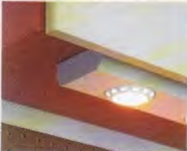
▲ Task Lighting. Lights mounted under the upper wall cabinets are ideal for detailed tasks.
